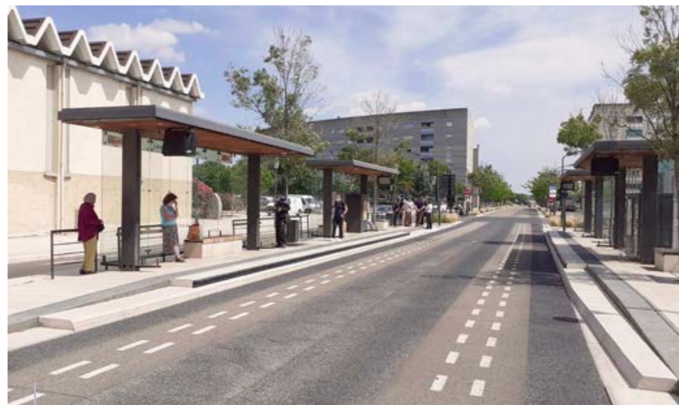
Station Trambus, à Nîmes
